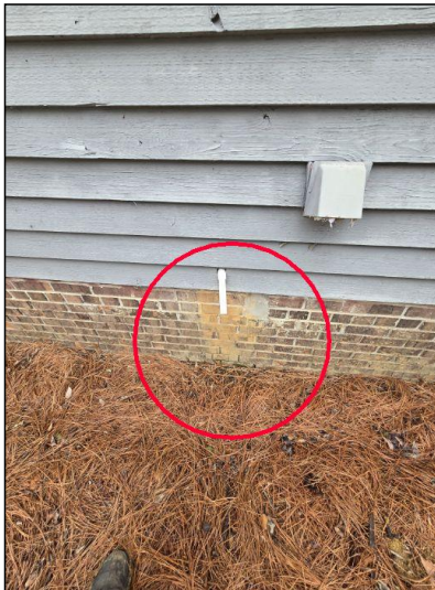
Water damage.
