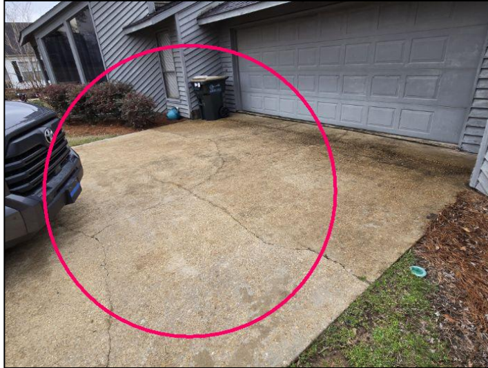
Small cracking.
