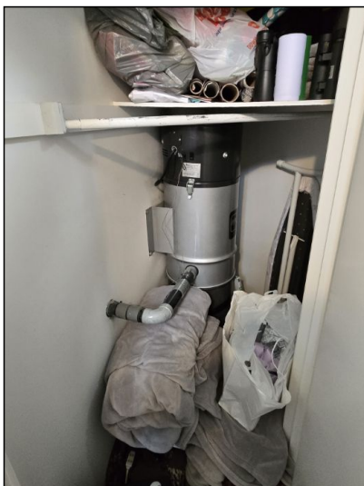
Central vacuum. Not checked due to blocked by owners belongings.
