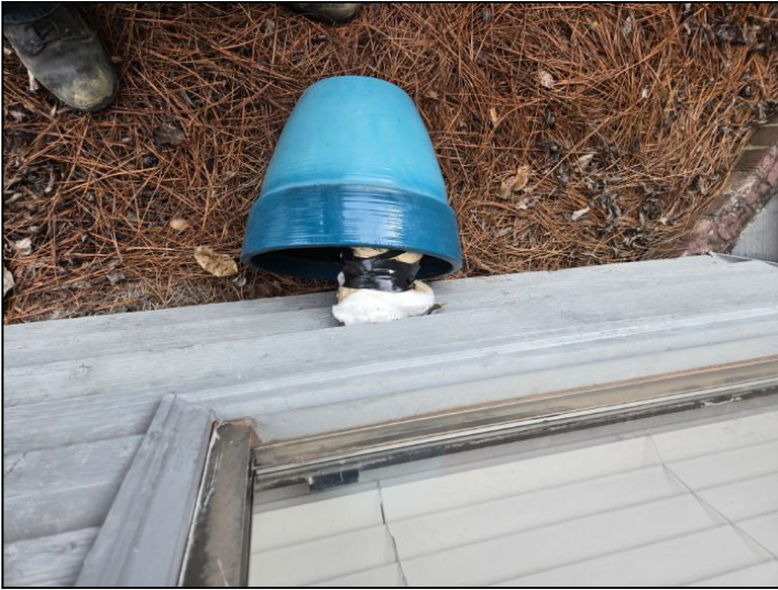
Located front of house. Unable to check due to covering. Located at front of house.
