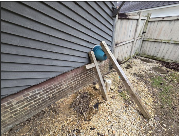
Located at rear of house. Unable to check due to winter coverings.
