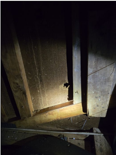
All holes to the exterior should be covered.
