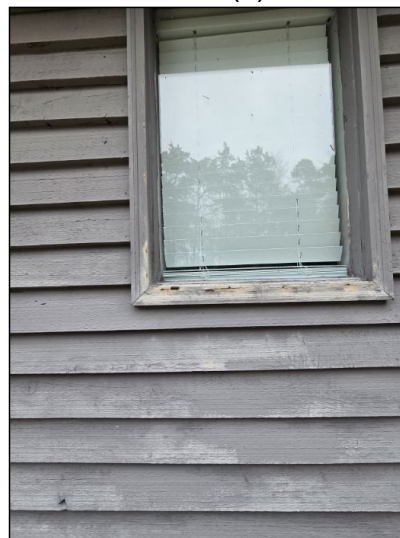
Deteriorated frame(s) at window(s)
