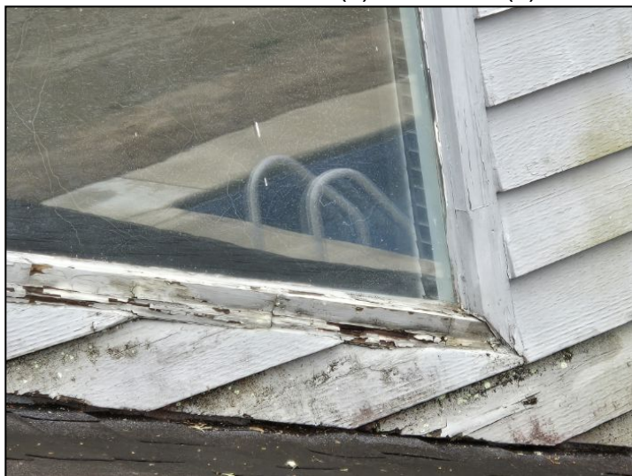
Deteriorated frame(s) at window(s)
