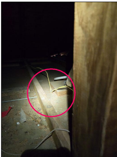
Connections made outside of a Junction Box, which is a potential shock or electrocution hazard.
