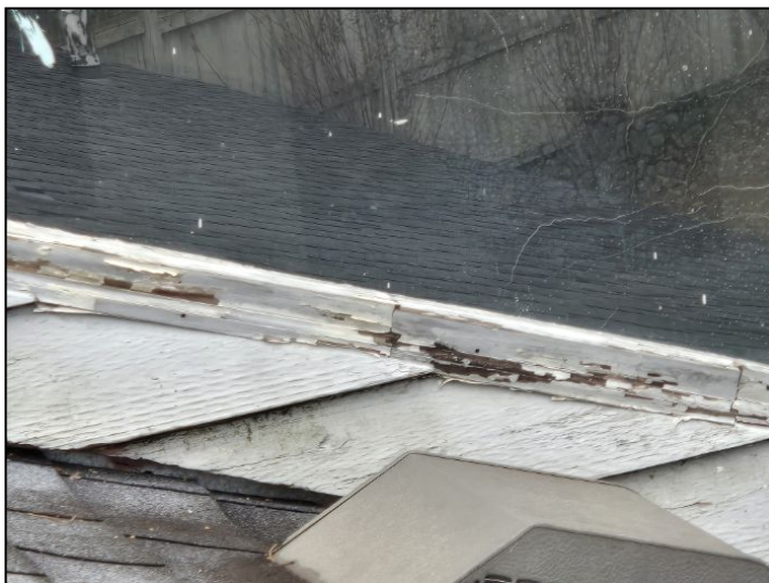
Deteriorated frame(s) at window(s)
