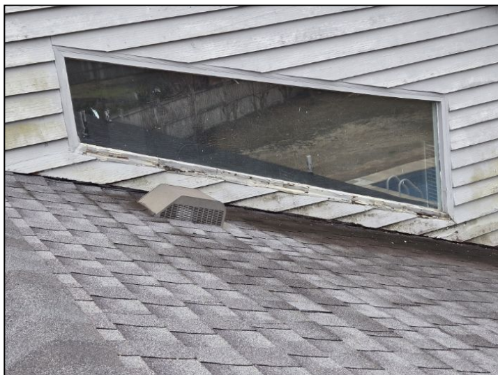
Deteriorated frame(s) at window(s)
